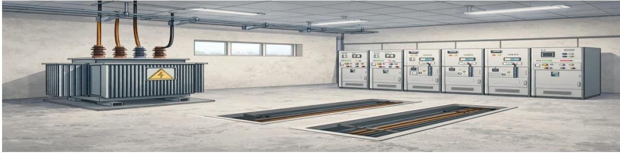
Fig. Indoor room with transformer, panels, and cable trenches.
