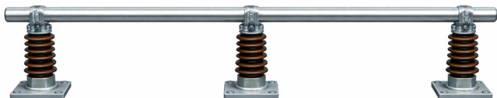
Fig. Straight aluminum pipe supported on insulators.
