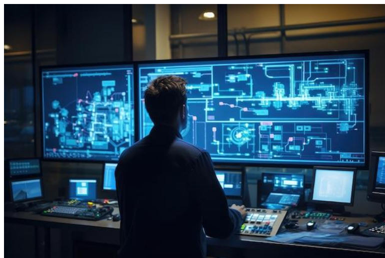
Control room with operator sitting at workstation
