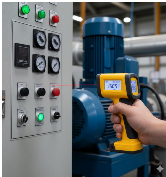
Fig. 1.4 - Handheld thermometer pointing at a motor panel.
